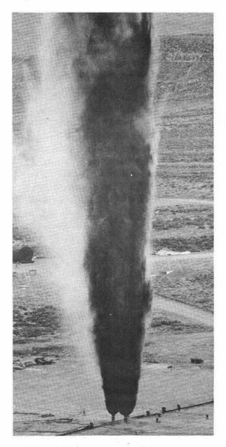
GASSES VENT through two well bores as nearly 7000 kg of slurry explosive rubblize an oil shale formation 60 m beneath the surface during an experiment near Rock Springs, Wyo. Sandia's Division 5734 conducted the experiment.
